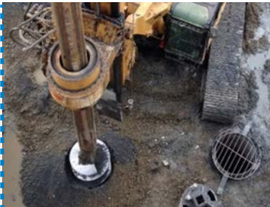
Bored Tension Pile: 35,000 m, Ø 1000 mm piles to the maximum depth of 15 m.
