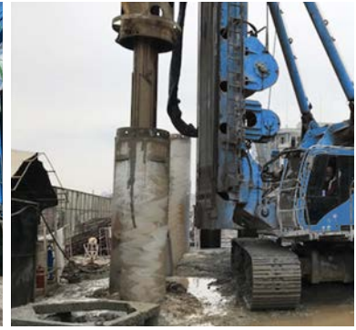
Secant piles: 7,000 m 2 , Ø 1000 mm piles to the maximum depth of 30 m.
