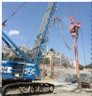
Vibro replacement: 100,000 m, Ø 800 mm columns to the maximum depth of 15 m.
