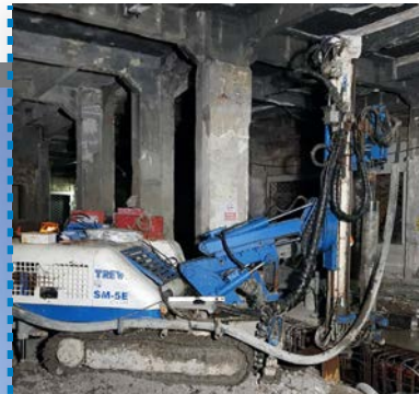
Underpinning micropiles: 2,000 m, Ø 250 mm micropiles to the maximum depth of 13 m.
